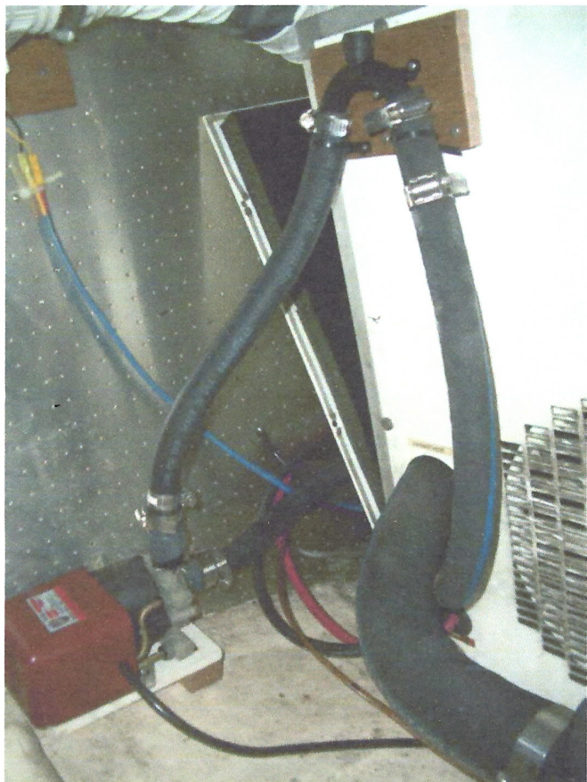
Figure 1 - March pump with anti-siphon loop and connection to generator
