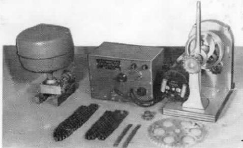
Model 11 Pilot with Compass Bowl Cover added. (A recommended accessory in damp installations.)
